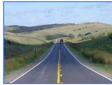
Asphalt Overlay - Callaway, NE
