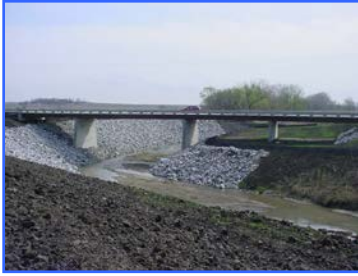
Bridge Structure - Syracuse NE
