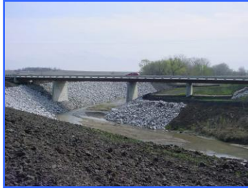
Bridge Structure - Syracuse NE
