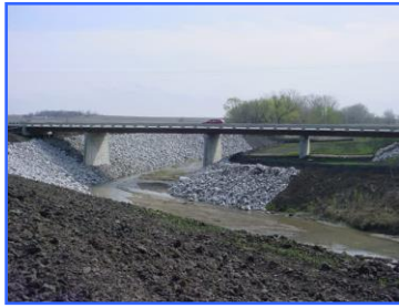
Bridge Structure - Syracuse NE
