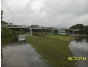
River Bridge – Orchard, NE
