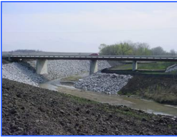
Bridge Structure - Syracuse NE
