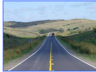
Asphalt Overlay - Callaway, NE
